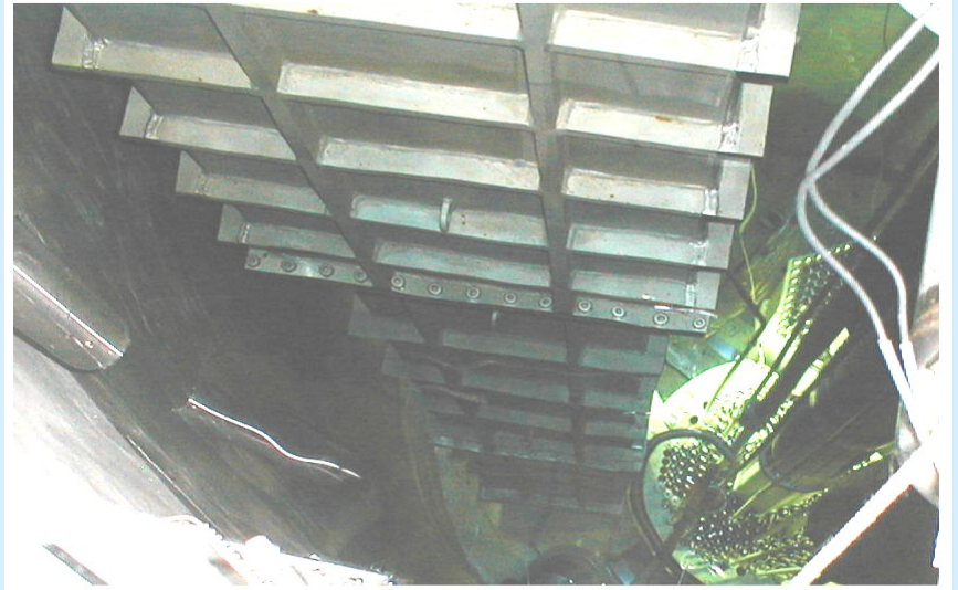
ACRR Tank View from West side
